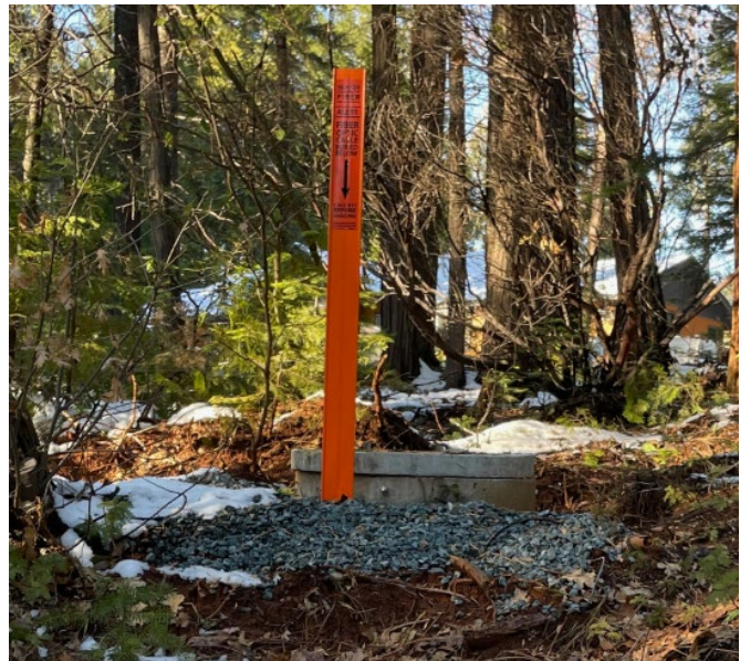
Figure 2: Nevada Company Fiber's new fiber optic installation.
