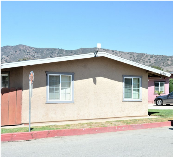
Figure 3: The San Jerardo Housing Cooperative (customer provided equipment)
