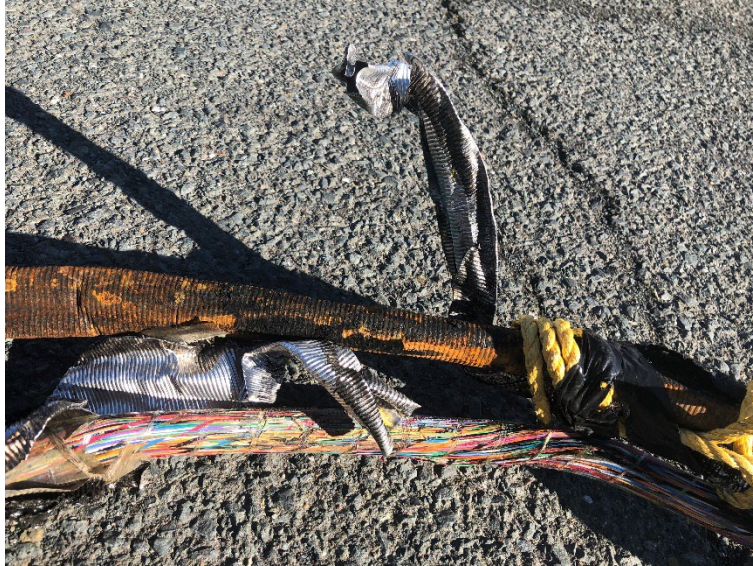
Figure 3: Damaged AT&T facilities
