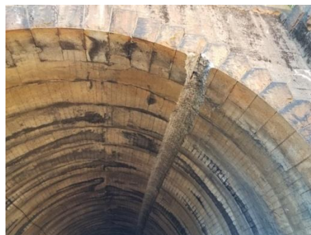
Groove in ceiling, UPRR Tunnel 34
