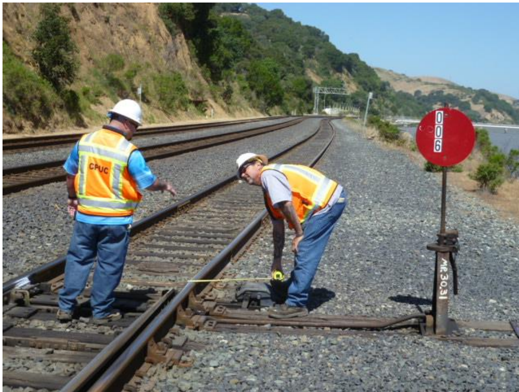
Track inspectors inspecting a switch on the UPRR
