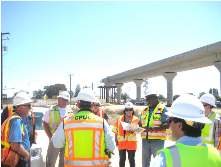
CPUC staff at the Cedar Viaduct construction site
