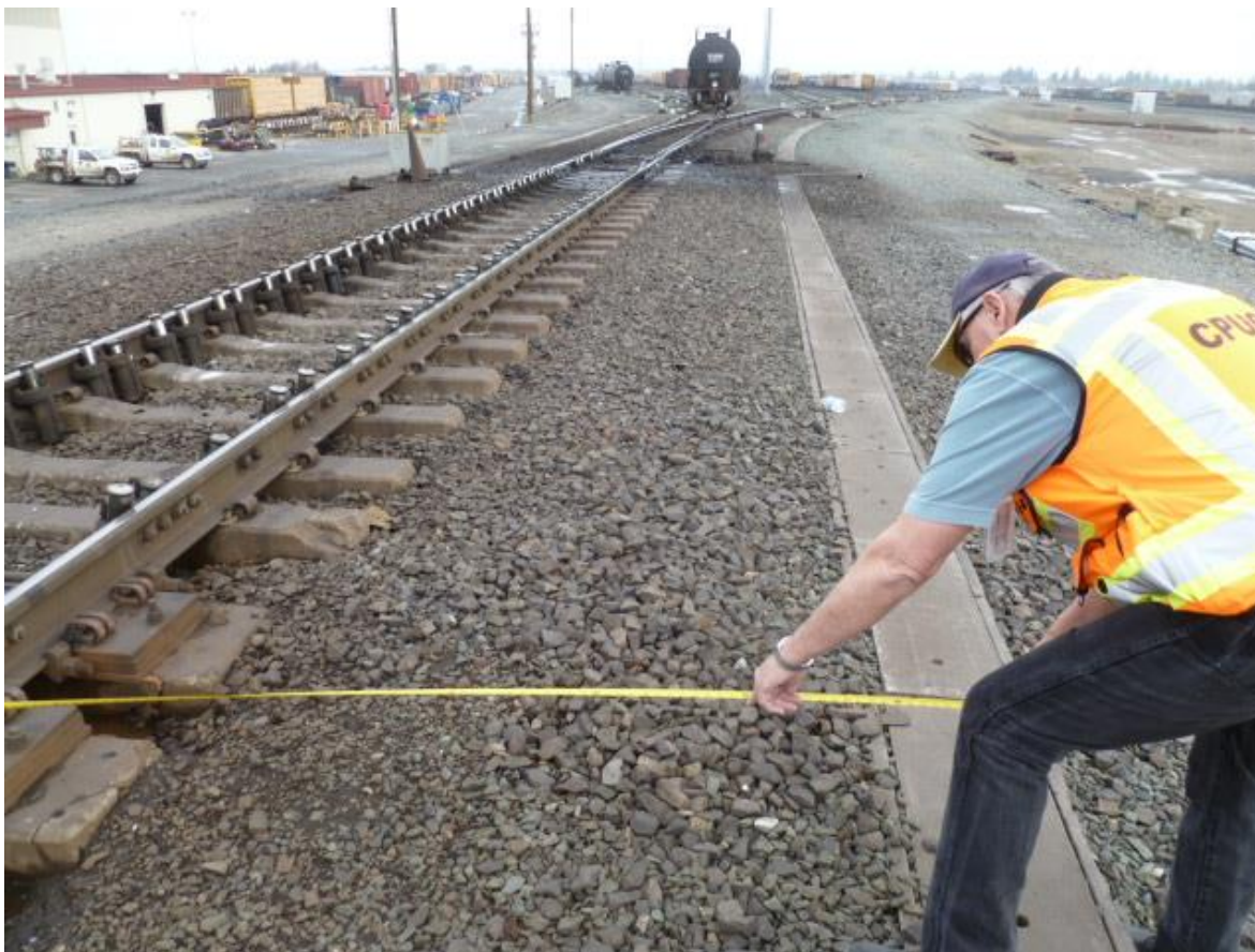
CPUC Inspector measuring walkway distance from track center
