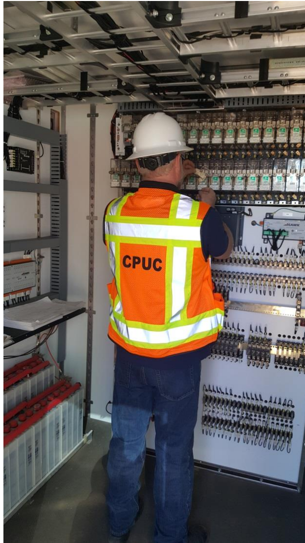
CPUC Signal and Train Control inspector, inspecting inside a signal house
