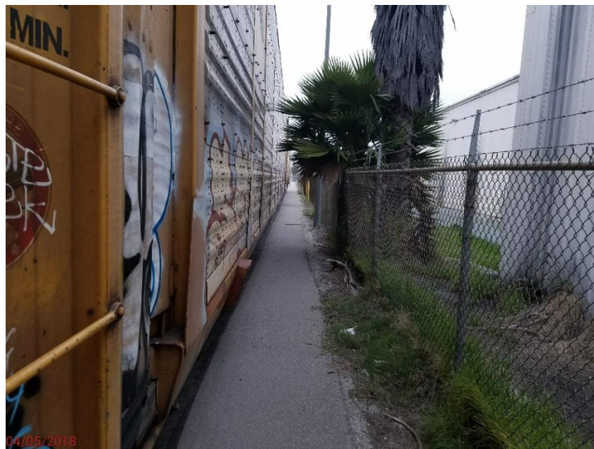
Vegetation impeding side clearance
