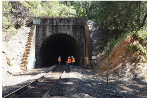
CPUC inspectors at UPRR tunnel #34
