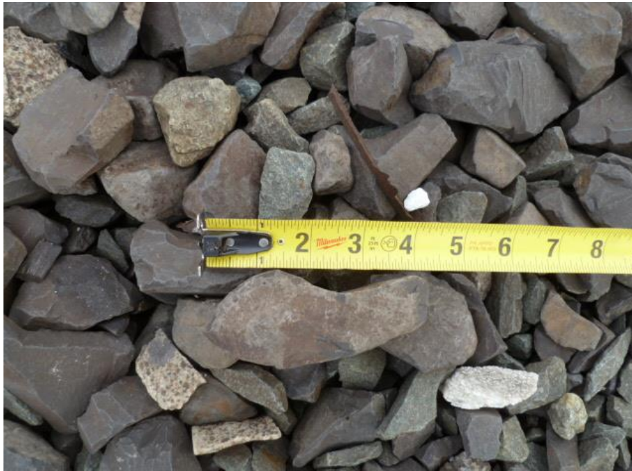
Oversized ballast, which creates a tripping hazard.
