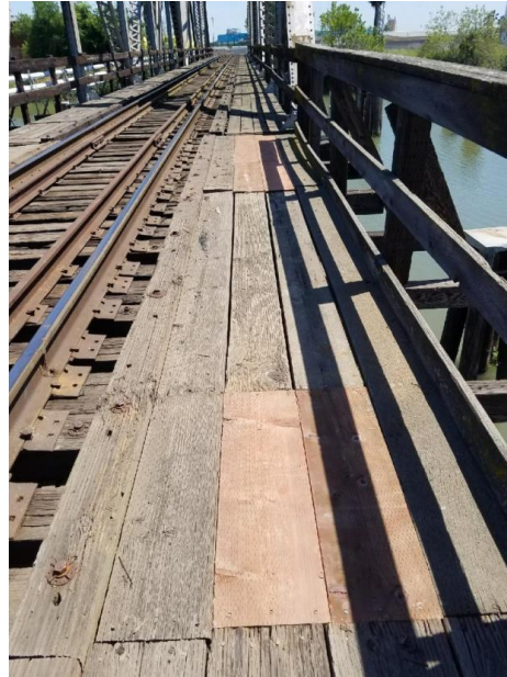
San Joaquin River bridge walkway after repair
