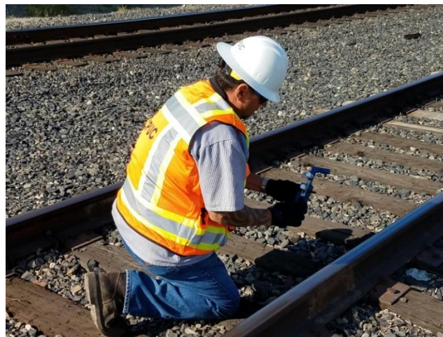
A CPUC inspector reading rail gage measurements
