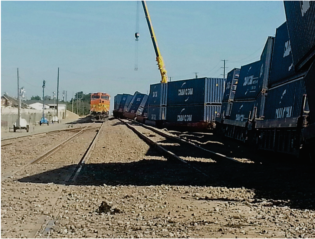
Double stack intermodal cars loaded with containers are being rerailed after the derailment Train was approaching on the main track to the right. The left track is the siding track
