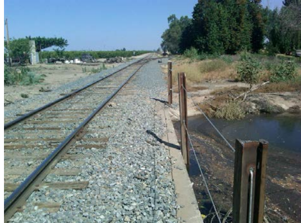
Follow up: safe walkway with handrails
