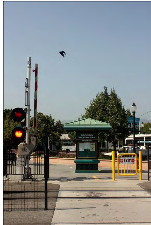
FIGURE 12 Example of Emergency Exit Push Gate in Combination with a Pedestrian Automatic Gate
