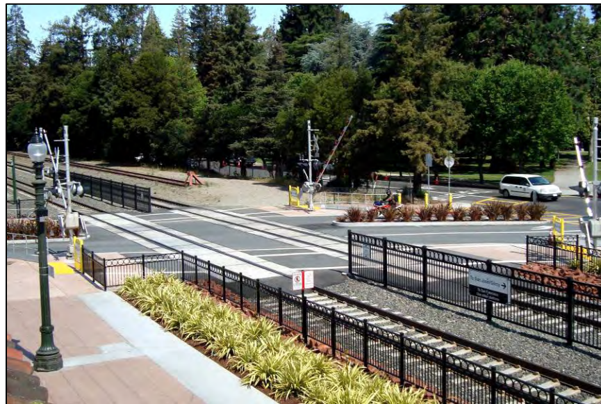
FIGURE 7 North Lane Highway-Rail Crossing: Northbound View After Improvements – May 2009
