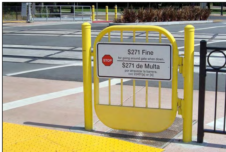
FIGURE 13 Fines for Misuse of the Emergency Exit Swing Gate
