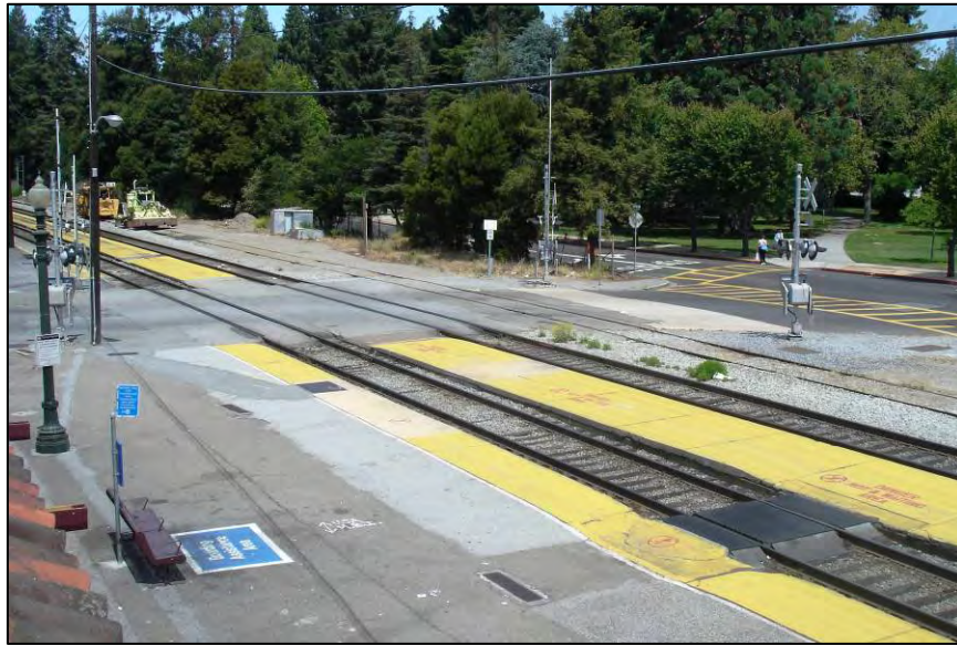
FIGURE 6 North Lane Highway-Rail Crossing: Northbound View Before Improvements – May 2007
