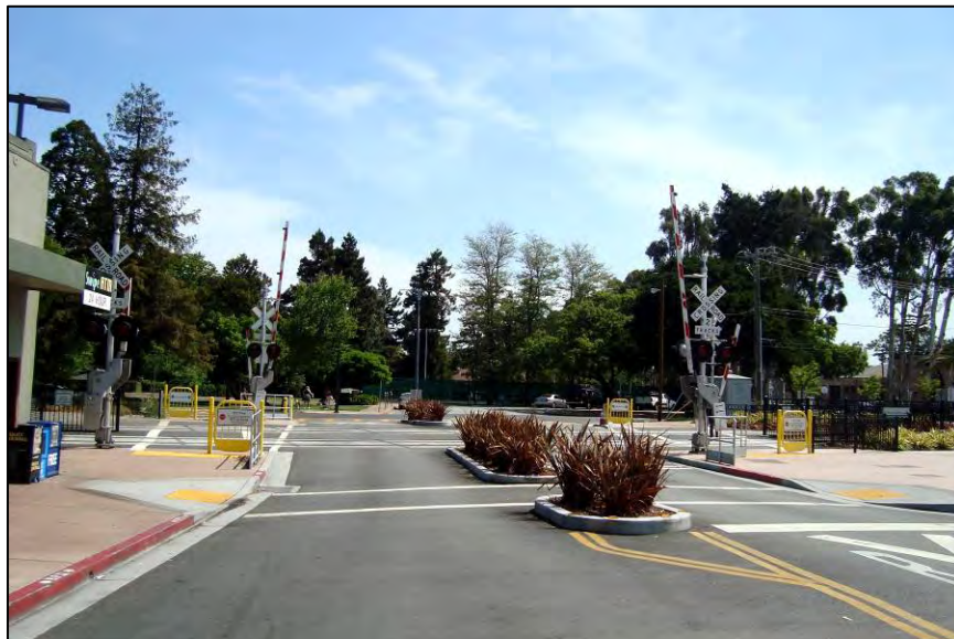
FIGURE 9 North Lane Highway-Rail Crossing: Eastbound View After Improvements – May 2009
