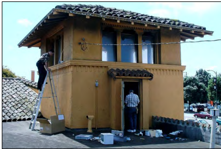
FIGURE 14 Installation of Video Monitoring Equipment
