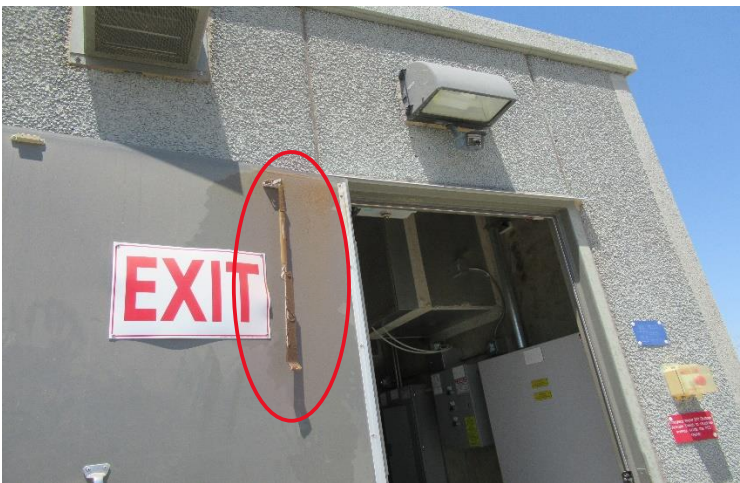
Figure 15: Inverter B10 02. The door auto closing mechanism was broken. This may have inverters exposed to dust, vermin and rainwater and result in the system failure and damage.
