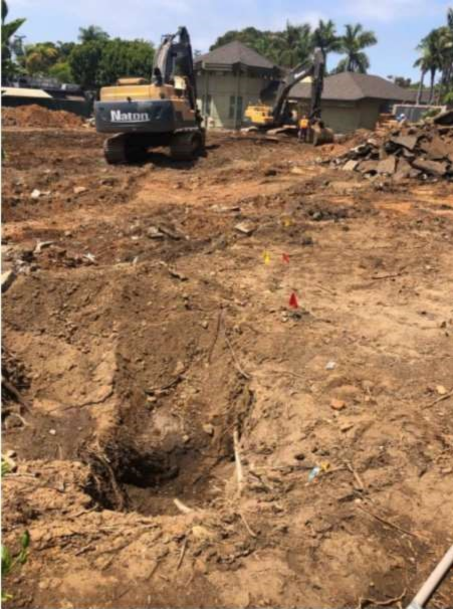
Image 8: Flags in area described on expired USA Ticket #A191060668 labeled Cable, Pipe and Leak.
