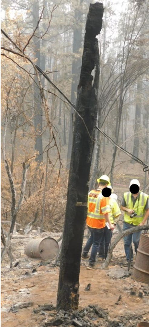
Figure 10: Remains of pole 434.
