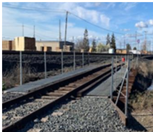
After: Vegetation cleared from bridge
