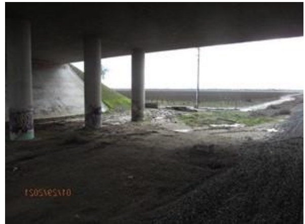
After: Encampment and debris removed
