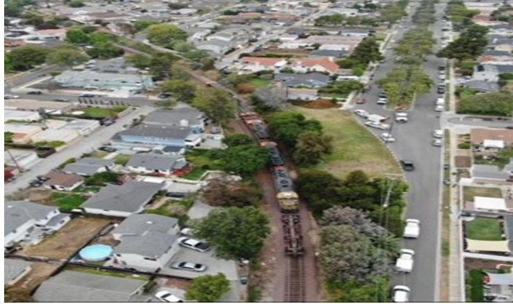
Overhead view of accident location 19
