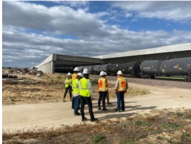
CPUC Commissioners and Commission staff viewing HSR viaduct, Wasco
