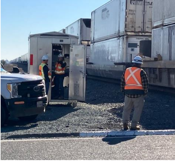
RSD Signal inspectors inspecting a signal box
