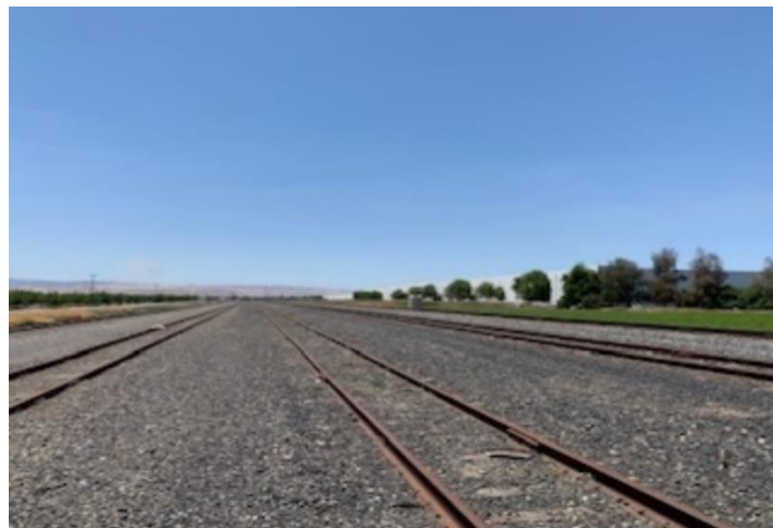
Tracy Yard after stored locomotives were removed
