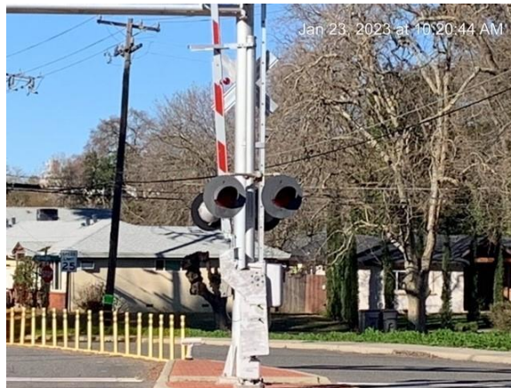
Signal light repaired
