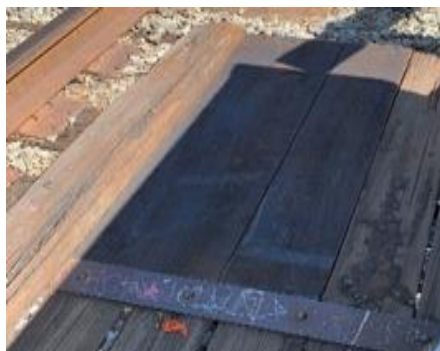
After: Walkway planks replaced
