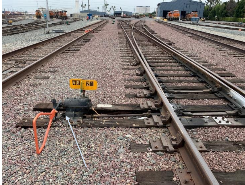
Repair track switch, not capable of attaching a locking device
