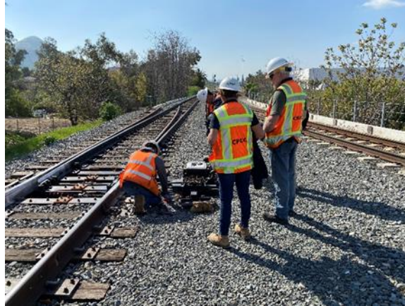
RSD Signal inspectors observing a power operated switch inspection
