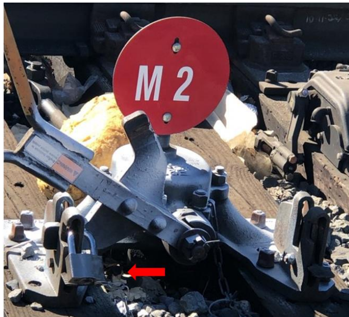
Switch equipped with lock after tracks were repaired
