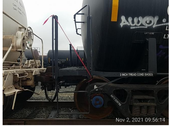
After: Warning tape placed on unsafe handrail until repairs could be made.
