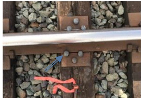
After: Spikes correctly installed
