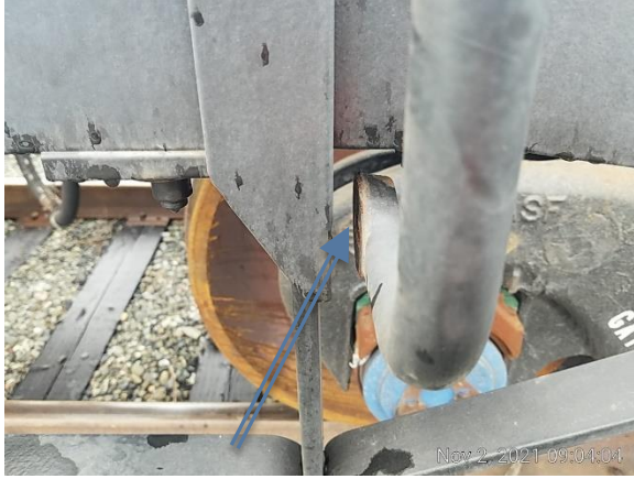
Before: Missing bolt on handrail
