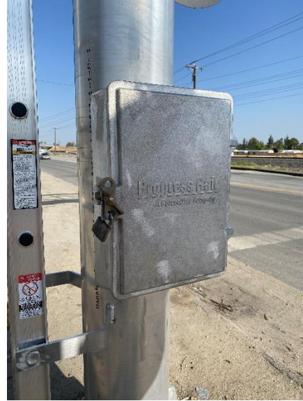
After: Junction box secured with padlock
