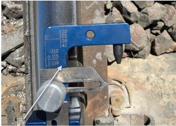
Measurement on gauge indicates 1" horizontal wear
