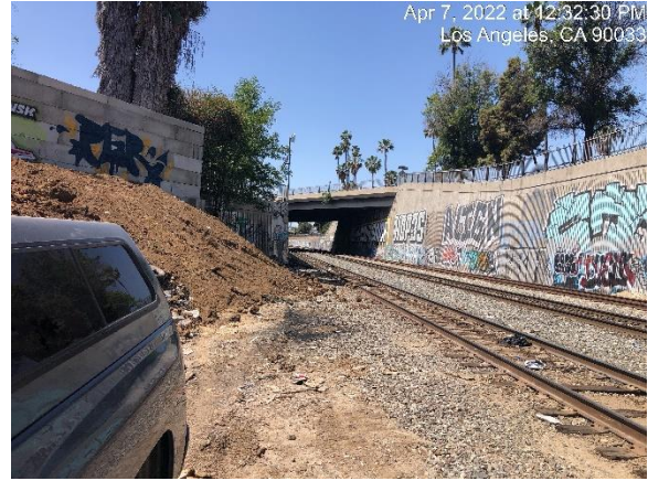
After: Debris removed from walkway surface
