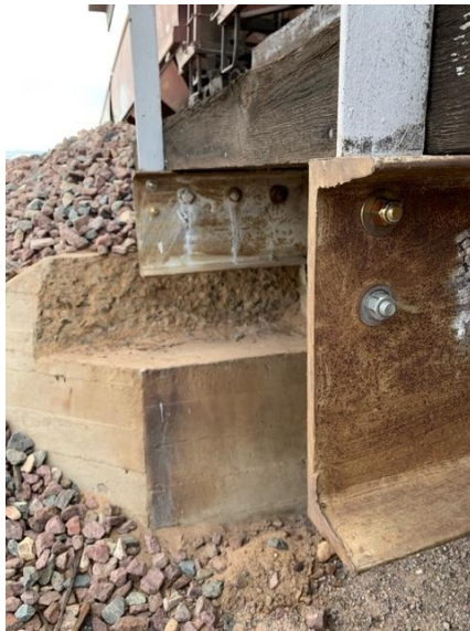
After: Bolts added to handrail
