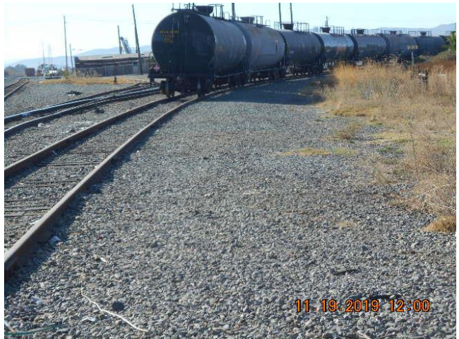
After: Debris removed from walkway
