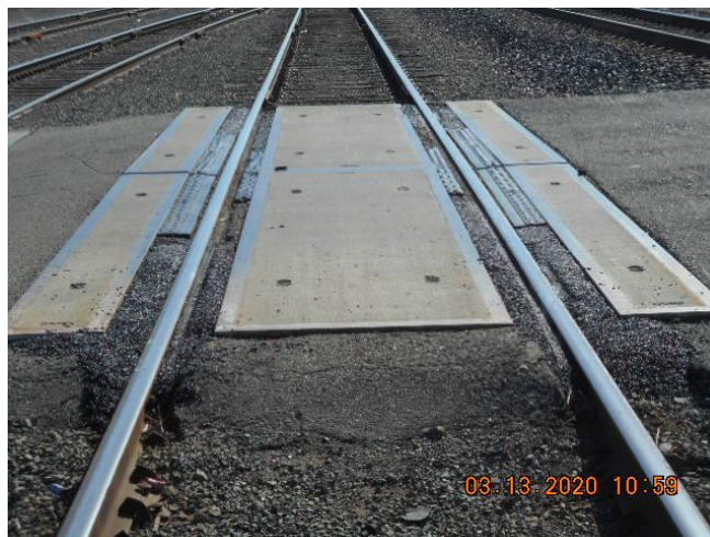
After: Approach grade repaired; now in compliance
