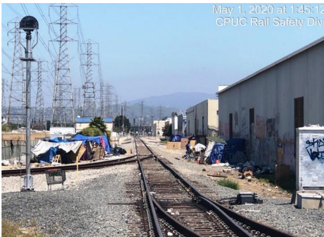
Before: Homeless encampment and debris near UPRR Anaheim tracks
