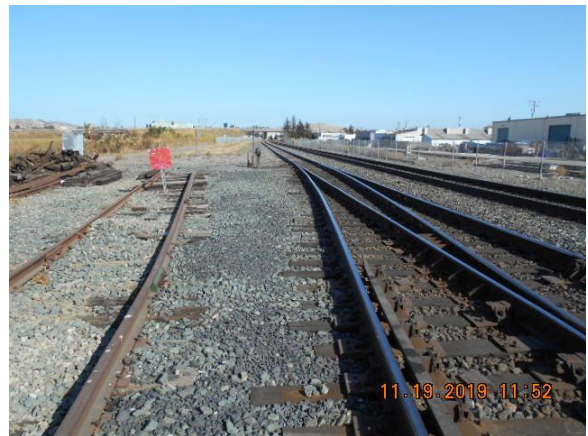
After: Ballast restored to GO 118-A standards
