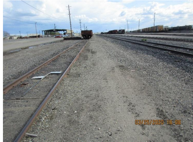
After: Blue Flag removed from walkway
