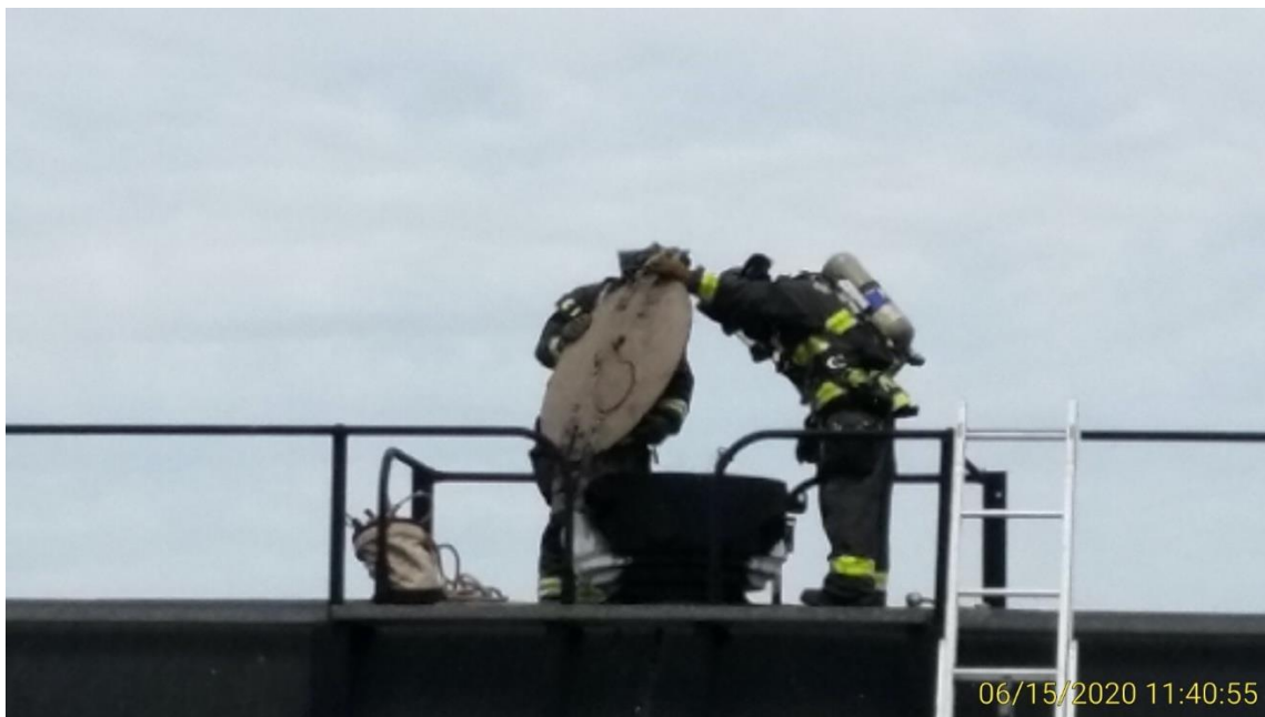
Roseville Fire Department in scuba gear checking inside dome for source of leak
