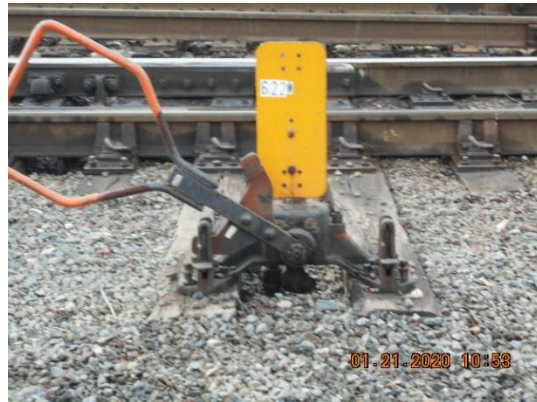
After: Ballast added; tripping hazard removed
