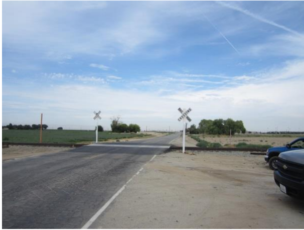
Before: Shafter Road looking east with passive crossing protection
