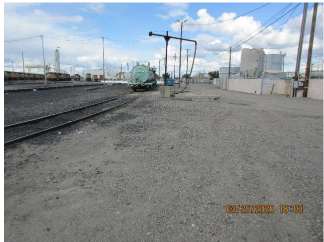
After: Locomotive cables removed from walkway
