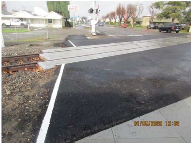
After: Crossing after repairs completed
