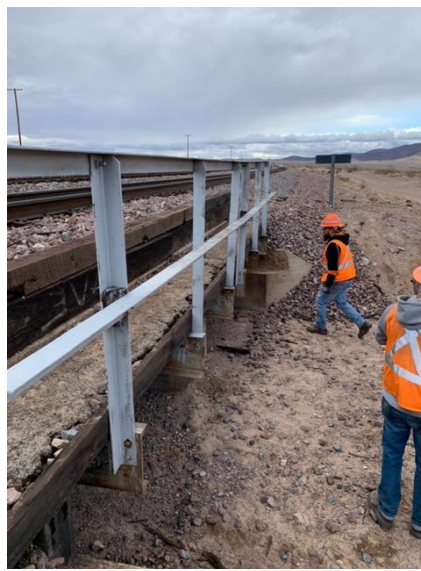
After: Handrail in correct position
