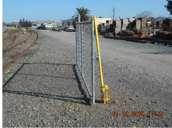
After: Gate restraint installed
