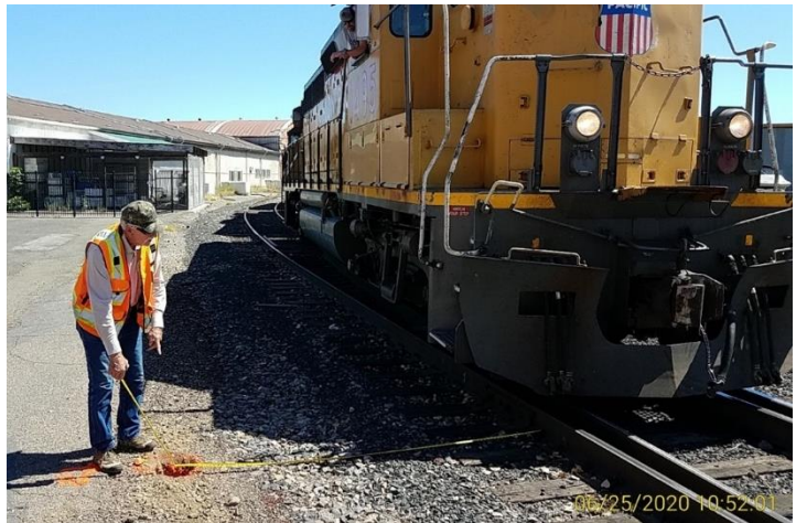
RSD inspector documenting defective walkway conditions (GO 118-A)
