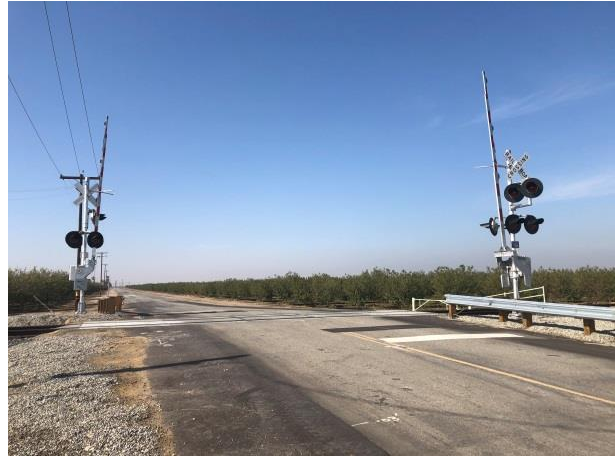
After: Shafter Road looking west with new active crossing protection installed
