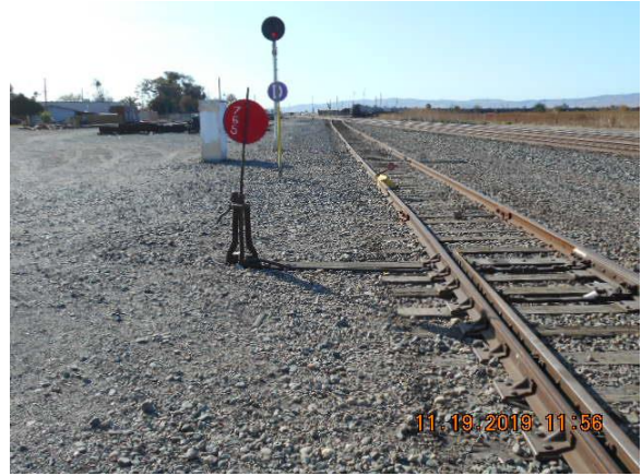
After: Angle bar removed from walkway
