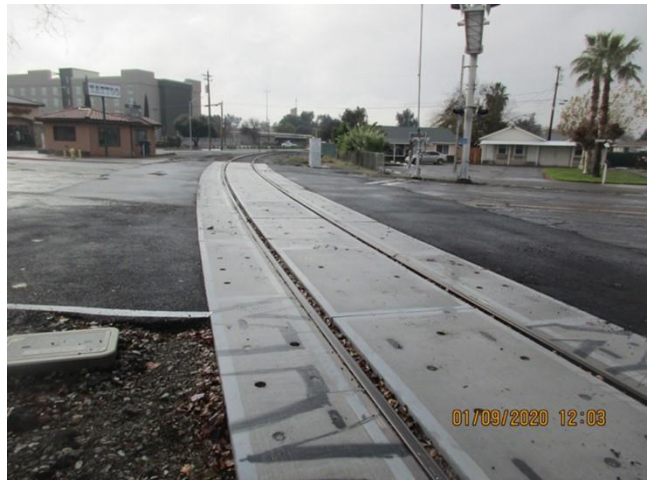
After: Crossing after repairs completed
