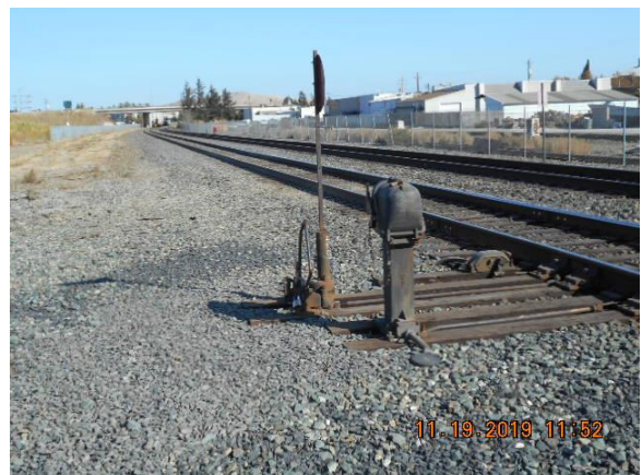
After: Ballast restored to GO 118-A standards
