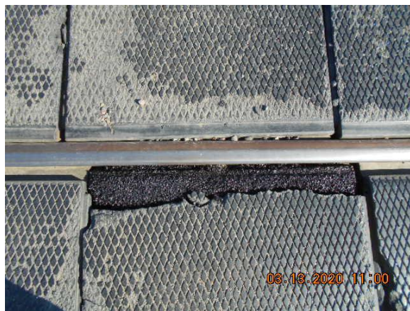
After: Flangeway gap repaired with asphalt; now in compliance
