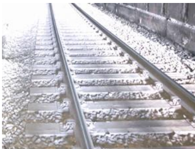
After: Clean ballast installed, drainage restored
