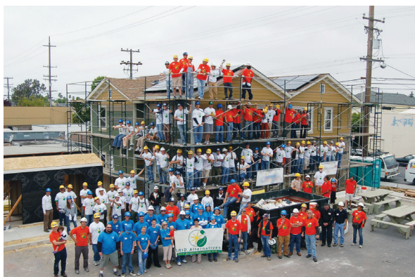
GRID Alternatives Solar Project for new housing development in Oakland, CA - October 2009
