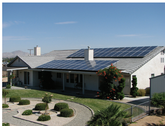
Desert Solar in Apple Valley, CA- July 2009-Solar system size 8.787 kW (photographer Don Jones)
