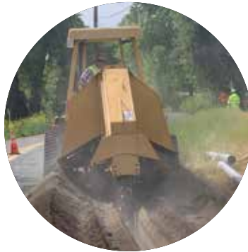
Alvah Group, Inc.: Undergrounding Fire Hardening
