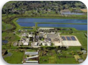
Waste Water Treatment Plant
