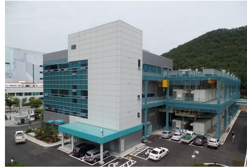
Busan Green Energy Project: 30.8MW, photo courtesy of Doosan
