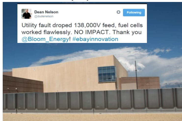
Data Center Utility Outage 4/16/15
